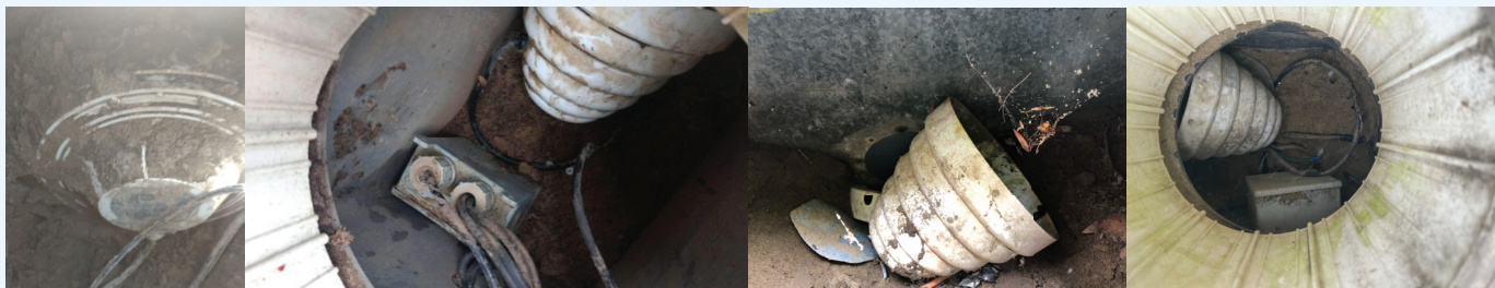
Note: Above are examples of boxes NOT cleaned and conditions of the lights.
